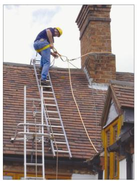
Constructed from user friendly 1/2" diameter, 12 strand polyester and polypropylene braided cover manufactured directly over a 1/4" diameter galvanised steel aircraft cable core. Aluminium compression fittings securely capture both steel cable core and the braided rope jacket.
